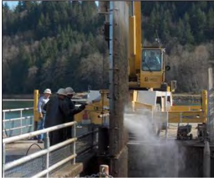
(louwered intake maintenance showing support structure and screens.)
