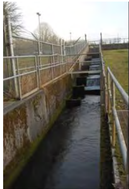
Attraction water flows into the creek from the fish ladder , whose purpose is
