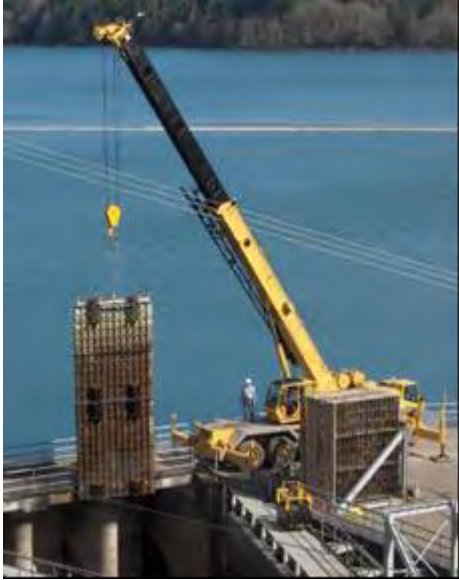
(louwered intake maintenance showing support structure and screens.)
