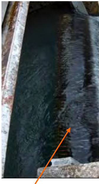
A finger weir at the holding pool assists in keeping fish contained until they are hand sorted.
