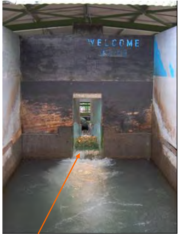
Flume entrance when attraction water cascades through the gate.
