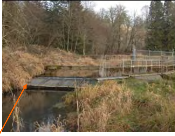
A barrier on Blue Creek at entrance of the fish ladder prevents fish from continuing upstream.
