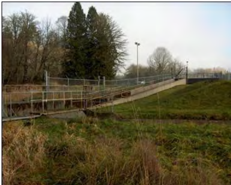
Attraction water flows into the creek from the fish ladder , whose purpose is
