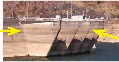
Spillway piers - side view
