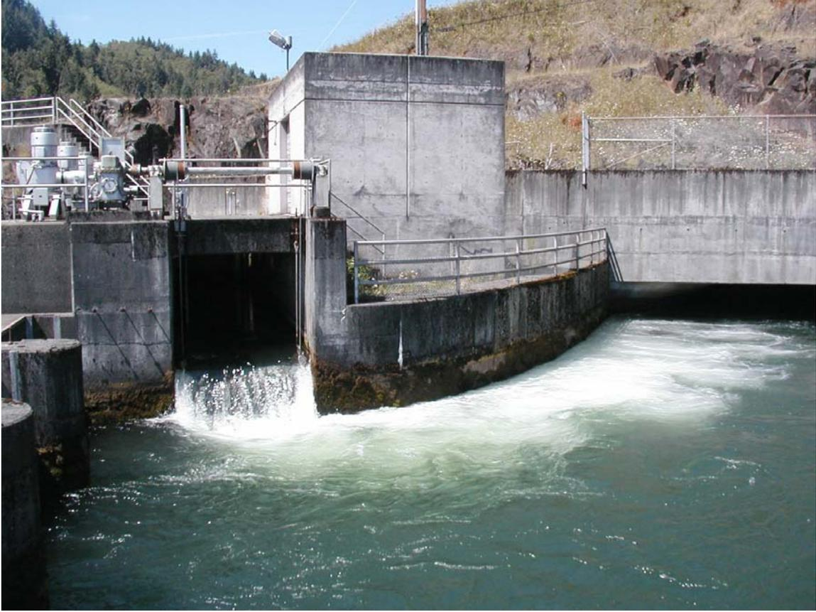
**Photo 10** - Bypass flow being pumped back downstream of the louvers.
