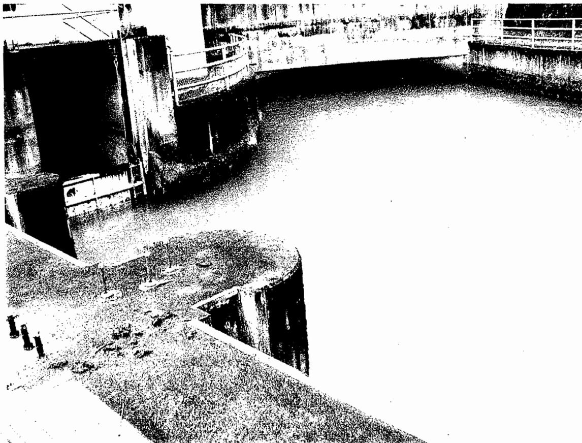
**Photo 8 – Secondary Dewatering Structure Pump Back Weir (far left) & Power Tunnel Entrance (center top)**
