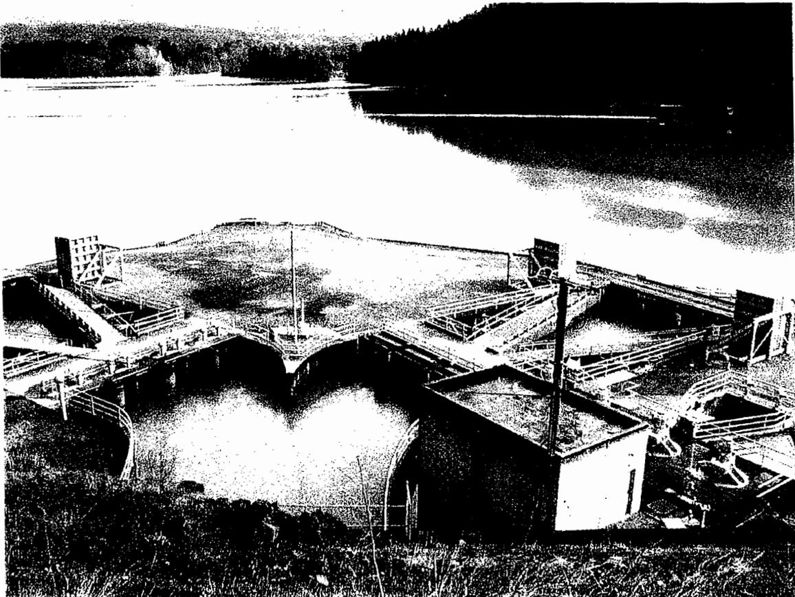
**Photo 2 – North (left) and South (right) Louvered Intake Bays**
