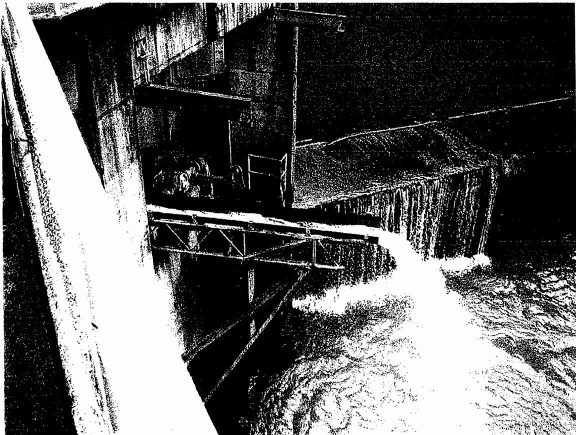
**Photo 12 – Smolt Bypass Discharge into Tailrace**
