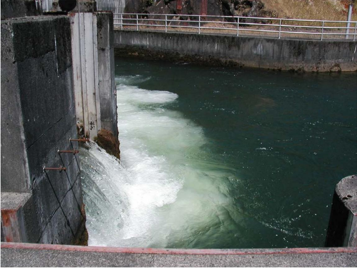
**Photo 11** - Close up view of bypass flow being returned to powerhouse tunnel.
