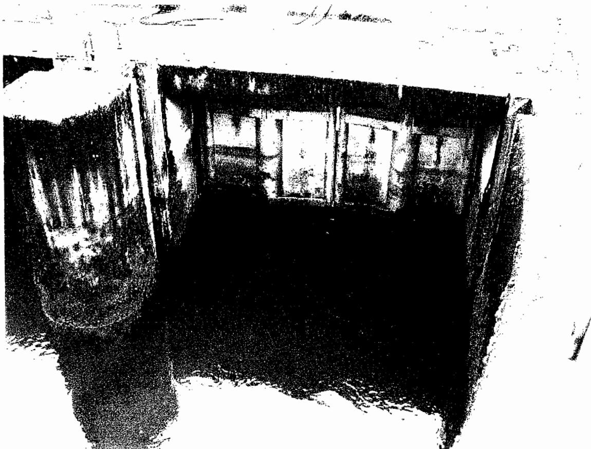
**Photo 13 – Wing Gates Closing North Intake Bay**
