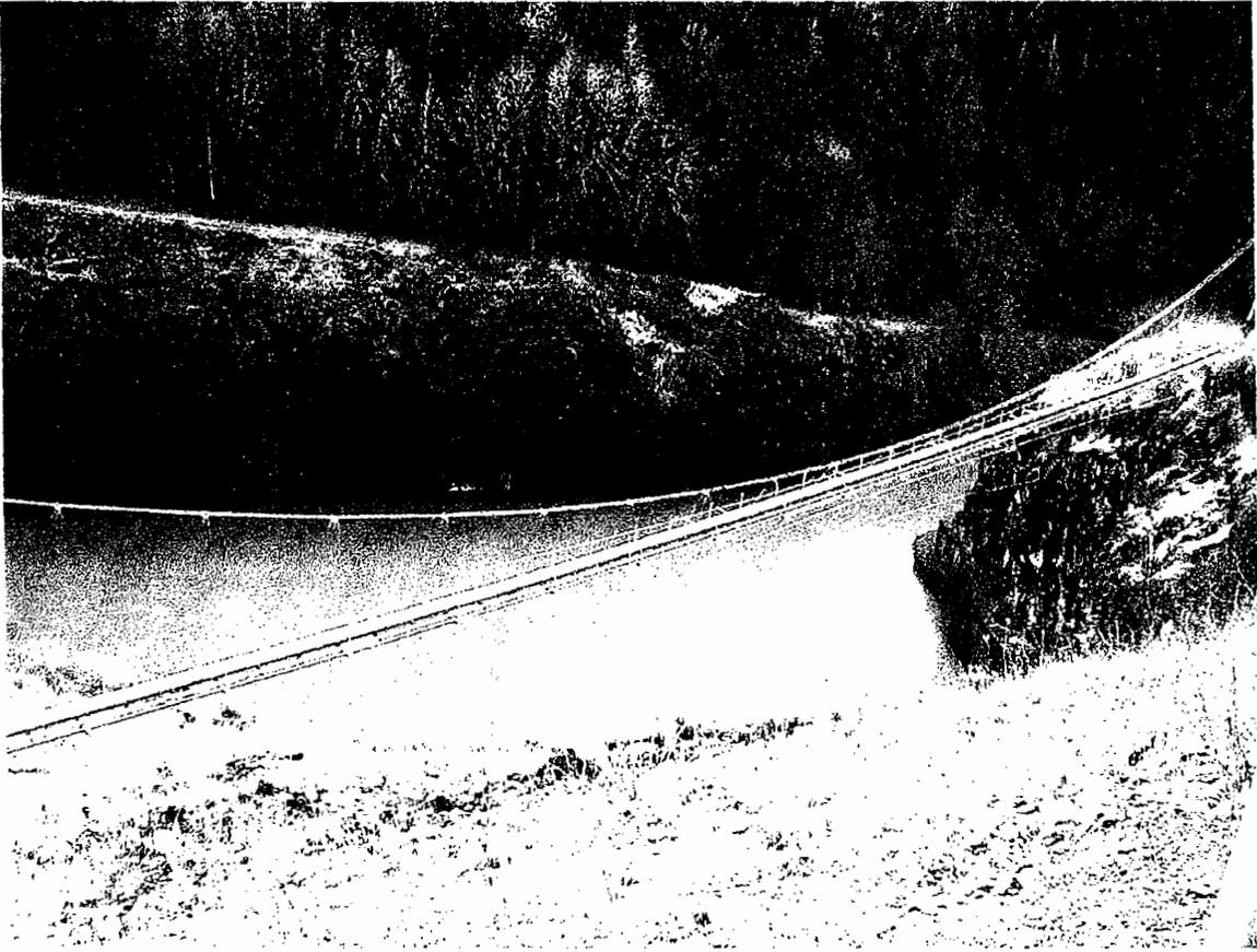
**Photo 11 – Smolt Bypass Pipe Leading to Powerhouse (beyond right side of frame)**
