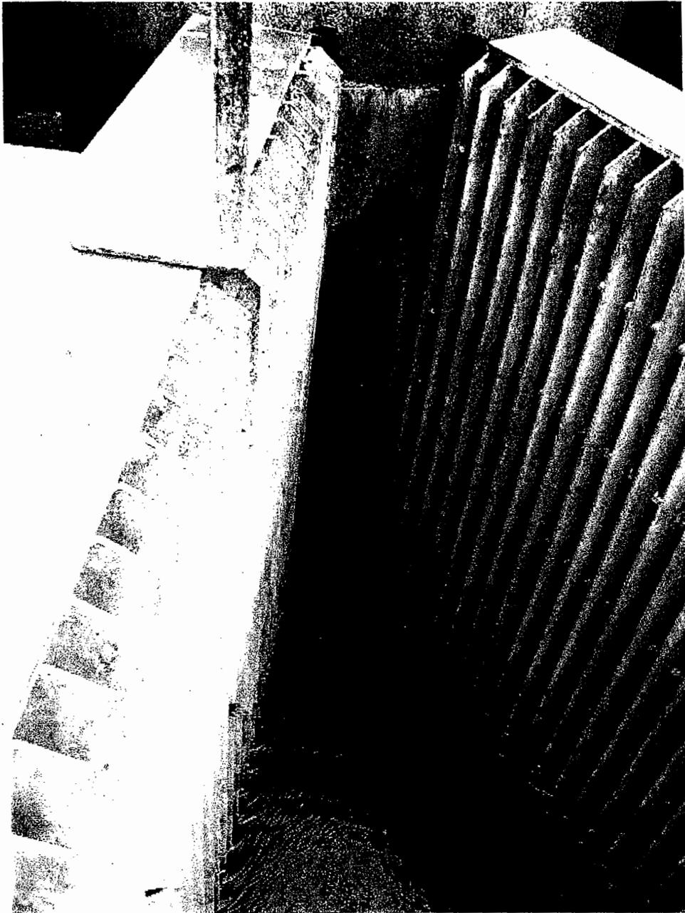
**Photo 4 – Bypass Entrance Slot and Louver Detail from U/S**
