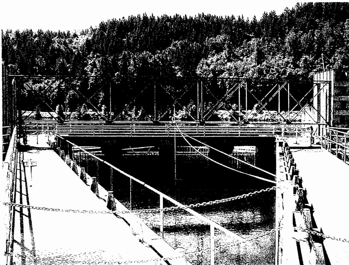
**Photo 14 – Truss Spanning Intake Bay & Used To Make Velocity Measurements**
