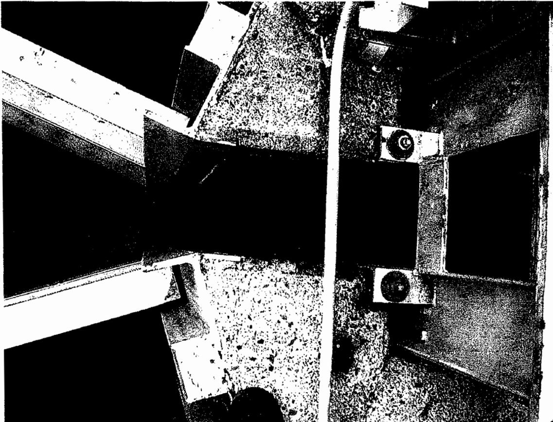
**Photo 9 – Secondary Separator Bypass Entrance Weir (flow from left to right)**
