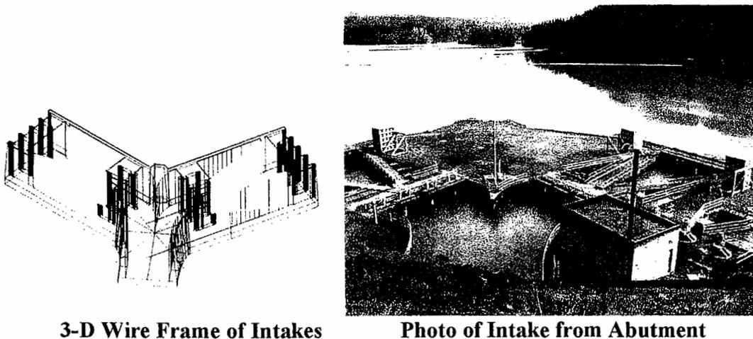
**Figure 1. North and South Louvered Entrance Bays of Intake Structure**
