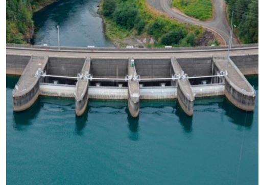
Mossyrock Dam's five spillway piers at full lake level
