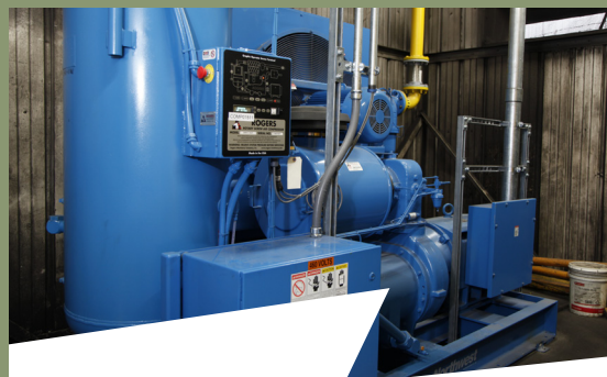
New variable-speed compressor reduces power input and airflow output to improve efficiency.
