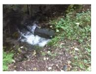
• There was an apparent cross connection between the spring collection manhole "blowoff" and the creek. The blowoff discharge was submerged and was isolated from the spring collection manhole by a single gate valve.
