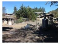
water. The Ozone Facility contains two ozone generators which are typically alternated in use. The plant uses pure oxygen to feed the generators. There are also two liquid oxygen tanks that are alternated in use. Ozone is injected into carrier water using up to three venturi injectors for each reactor: two 6-inch venturis and one 4-inch venturi. The original contract for the installation of the injectors specified a minimum ozone transfer rate of 95% to
