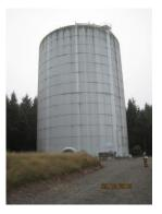
good condition. The roof is accessed annually and in response to intrusion alarms. The roof was last accessed in April. It was reported that the screened vents and hatches were in good shape.
