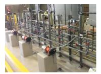
had caused a low chlorine episode a month ago when flow looped back through a peristaltic pump that had recently been moved. The flow meter indicated proper flow to the injection point but it was not able to detect that some of the flow was looping back into the system through this pump. Minimum CT requirements were reported to have been met by taking ozone CT into account. Repairs have been made including installation of check valves to
