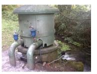
• There were unprotected openings into the pump wetwell between the cistern lid and the cistern itself (pictured at left). These openings have since been eliminated by the time of the report.
