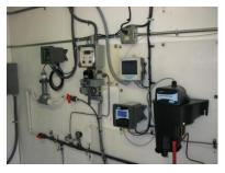
center building in the city. The turbidimeter (1720 E) is cleaned every week. It was unclear whether it has been calibrated recently. *It is recommended that the turbidimeter be recalibrated once per quarter.* There is an autostart generator on-site for power outages. At the time of the survey the following values were noted:  $Cl_2 - 1.4 \text{ mg/L}$ , Turbidity – 0.89 NTU, pH – 7.95, Temperature – 17 °C. The facilities were in excellent condition.
