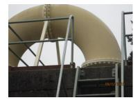
There is an emergency blow off at the north end of the reservoir site that allows direct access to PL1 (pictured at left). *The blowoff is covered by a wide mesh grate which must be protected by a finer mesh screen.* The hatch drains were in good condition and have proper drainage. *The hatch drain discharges should be covered with a fine mesh screen. This is true of all of the at grade reservoirs.*
