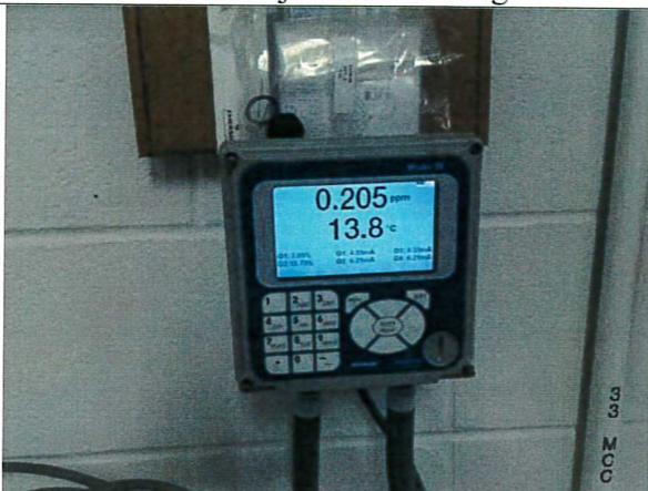
Ozone Sample Station 1 Analyzer Reading
