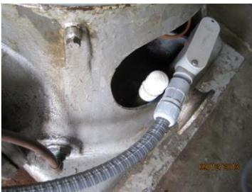
Wells SE#11 and SE#11A do not have vents and it appears that it would be difficult to install them. Like the other wells it does not appear a CT of 6 is provided to nearby customers who receive water from the well. There is a chlorine analyzer on site and at the time of the survey the free chlorine residual in the distribution system was 0.56 mg/L.
