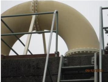
There is an emergency blow off at the north end of the reservoir site that allows direct access to PL1 (pictured at left). **The blowoff is covered by a wide mesh grate which must be protected by a finer mesh screen.** The hatch drains were in good condition and have proper drainage. **The hatch drain discharges should be covered with a fine mesh screen. This is true of all of the at grade reservoirs.**
