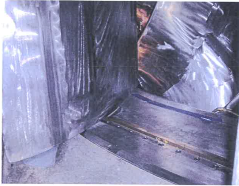
Figure 12: Lower Gate-End Seal with Wicket Gate in Open Position
