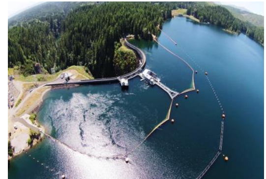
Floating Juvenile Fish Collector at Cushman Dam No. 1
