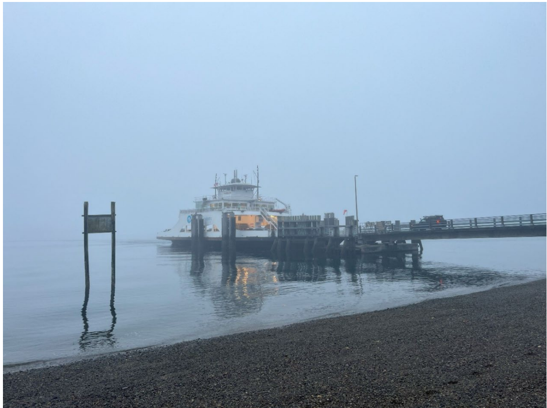
Figure 4. Ketron Island Ferry Terminal
