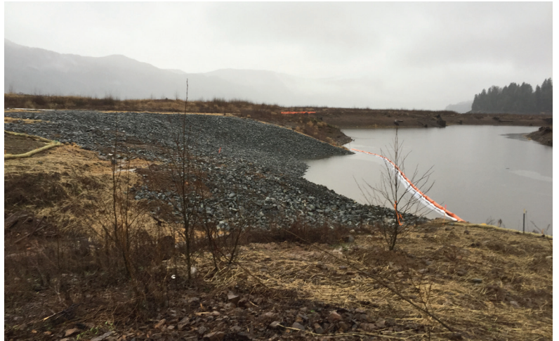
Tacoma Power recently completed this cap of the Kosmos Flats oil seep.
