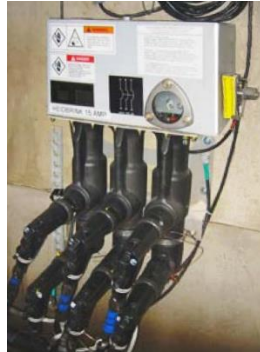
Figure 4 Fault Interrupter
