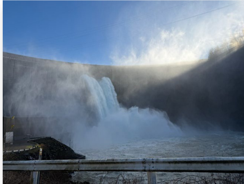
Cowlitz Hydroelectric Project – Mossyrock Dam Spill
