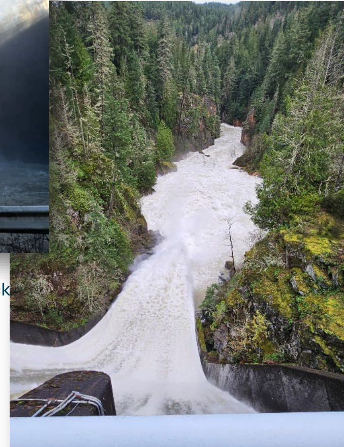
Nisqually Hydroelectric Project – LaGrande Dam Spill
