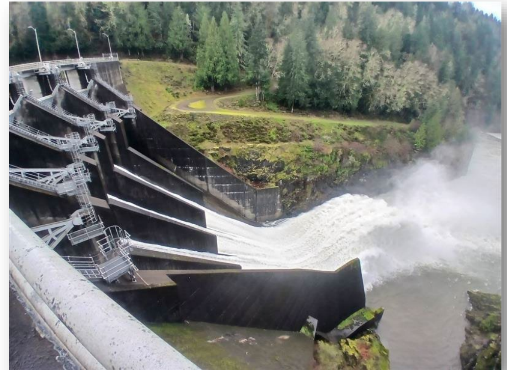
Cowlitz Hydroelectric Project – Mayfield Dam Spill
