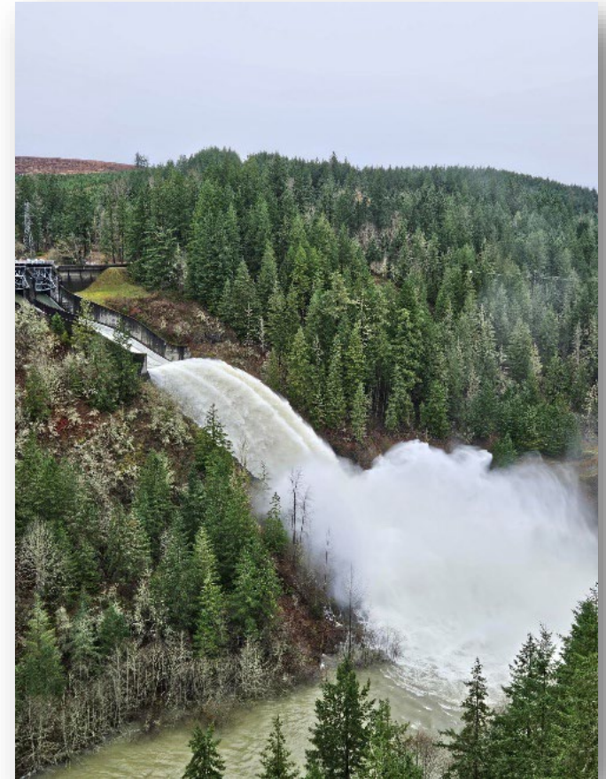
Nisqually Hydroelectric Project – Alder Dam Spill
