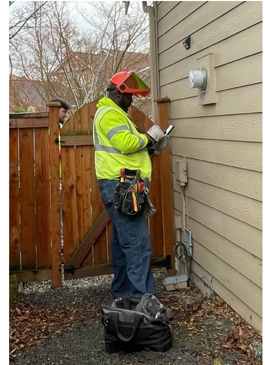
Final electric installed by vendor (03/20/25)
