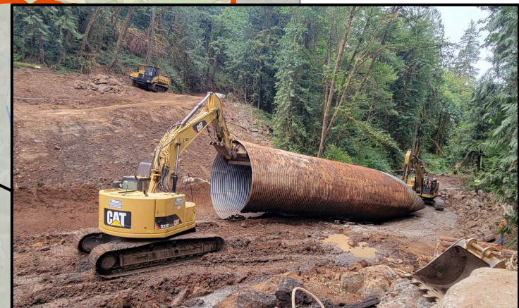
Photo from the Cowlitz Indian Tribe – culvert removal in Ostrander Creek
