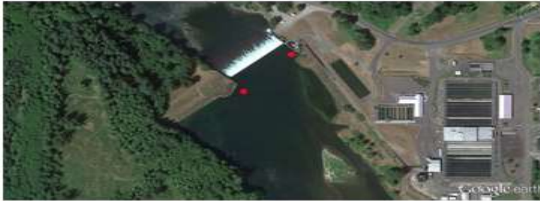
Barrier Dam (RM 49.6) Survival Detection Site 2
