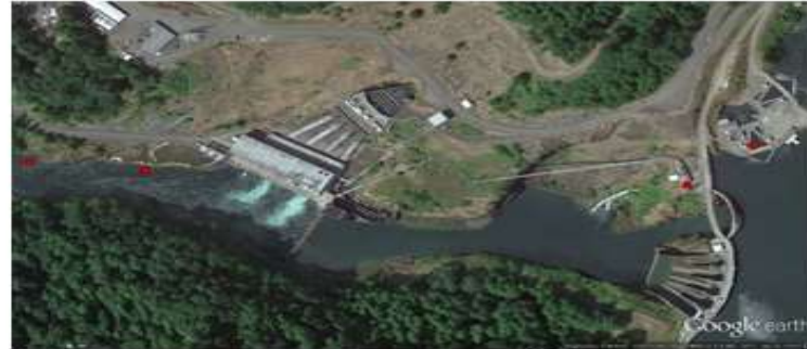
Mayfield Dam (RM 52)
