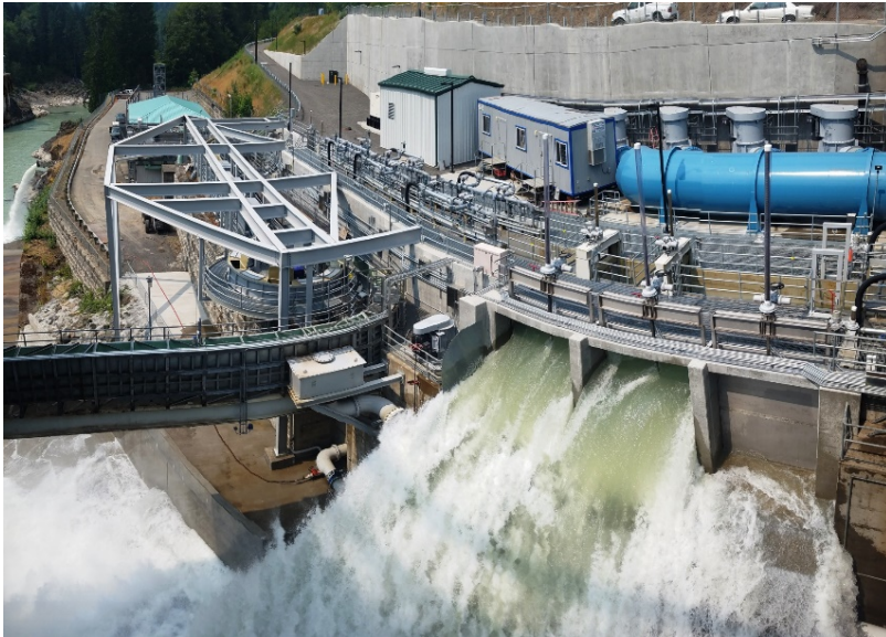
Cowlitz Falls North Shore Collector
