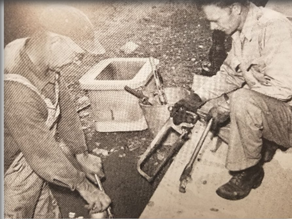
Installing new meters - at last. The $1.27 million installation program began in April 1954 and was completed 13 months later
